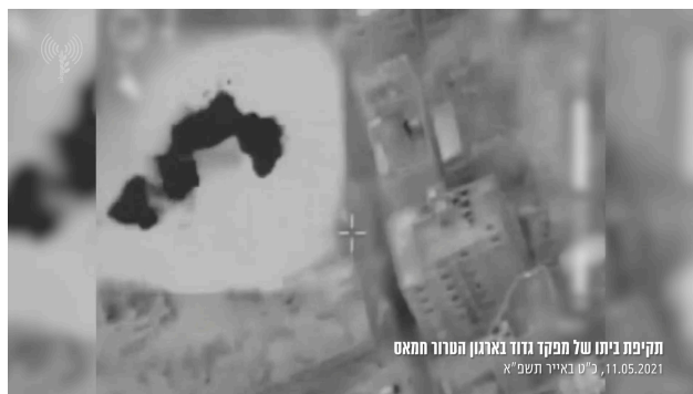
Figure 2: Image captured from the video shared by the Israeli Air Force showing the destruction of the top floors of the apartment building
